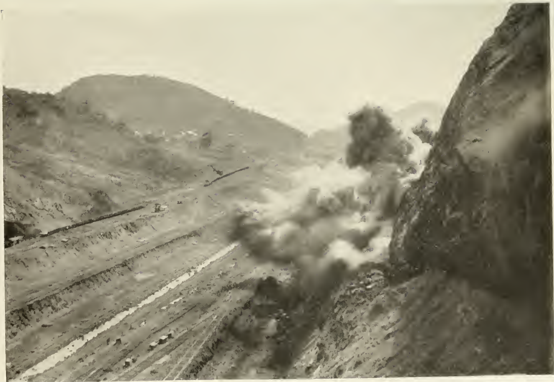
CULEBRA CUT AT CULEBRA; VIEW LOOKING SOUTH; BLASTING ROCK ON CONTRACTORS' HILL, JANUARY, 1912.
