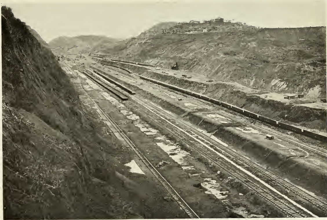
A SECTION OF THE GREAT CULEBRA CUT, JUNE, 1912.
