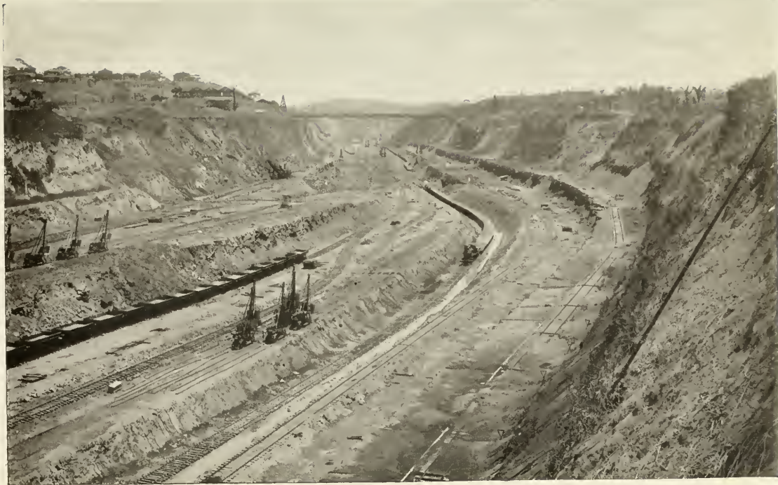
CULEBRA CUT, LOOKING NORTH FROM A POINT JUST SOUTH OF THE EMPIRE SUSPENSION BRIDGE, MAY, 1912.
